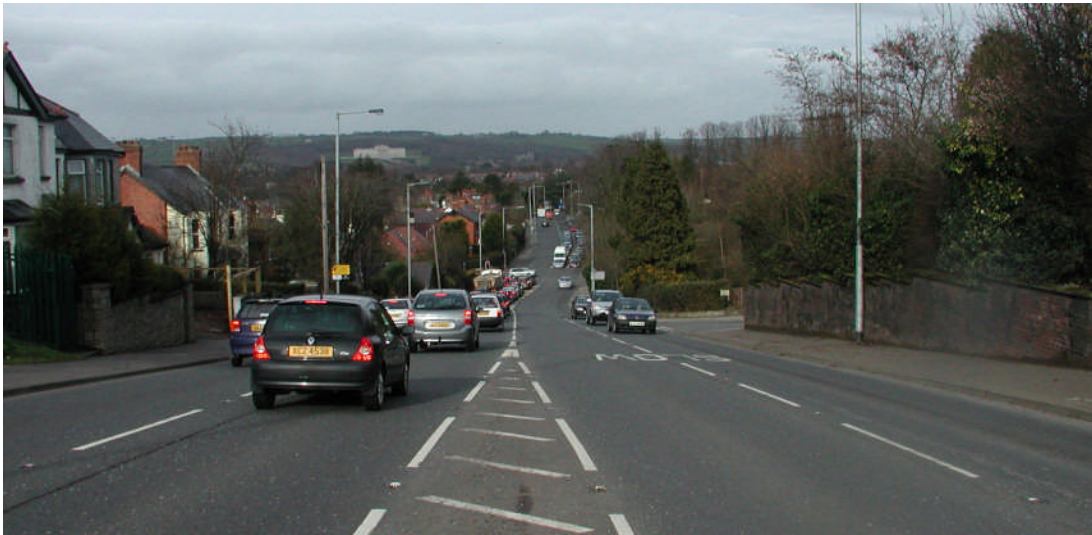
A55 Knock Road eastbound (existing)
